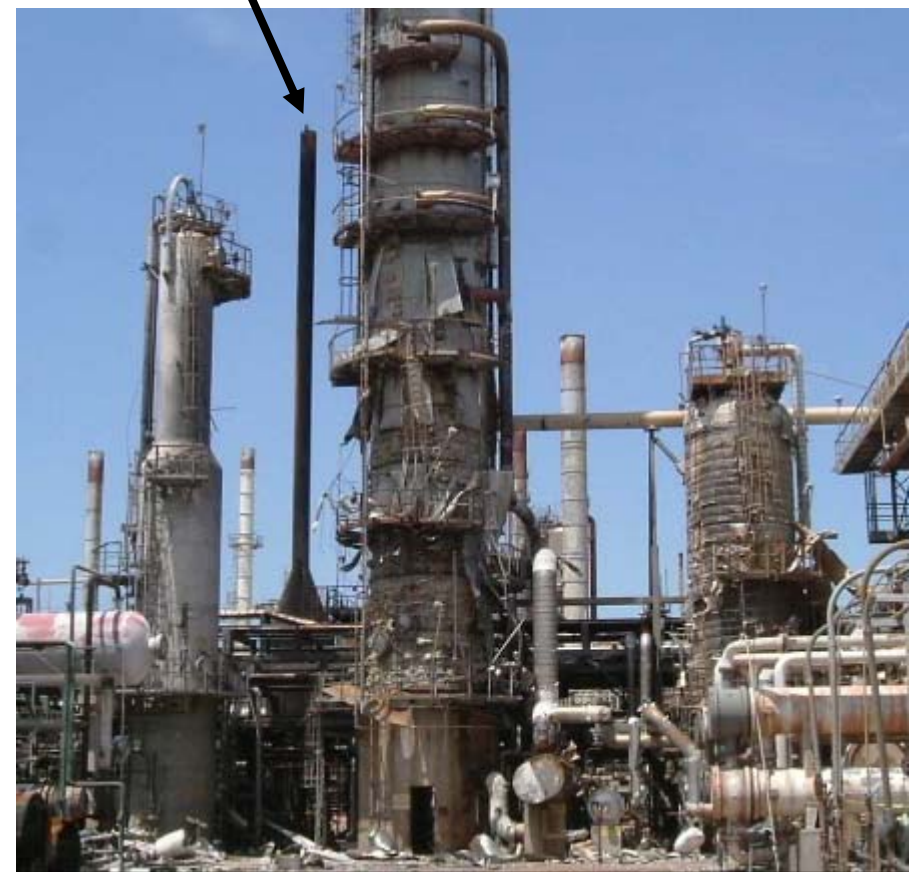
Blowdown Drum Stack
