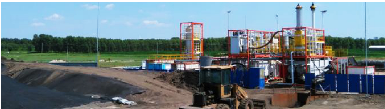
Fig. 5—Picture of the job site.
