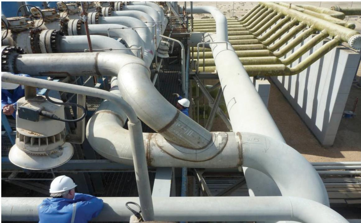
**Fig. 2—Seven blowdown 16-in. branches connected to 20-in. header.**
